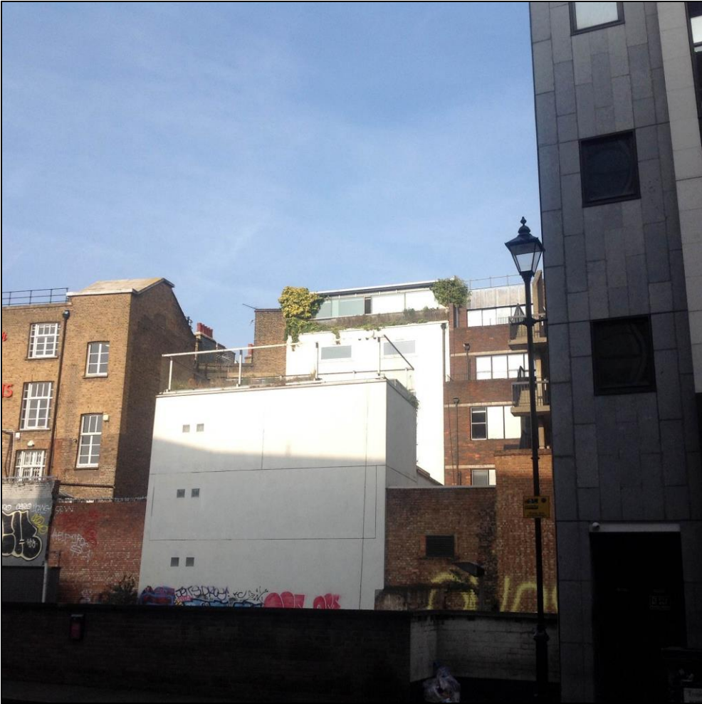
Image 6: View of adjoining buildings to the rear of the site.
