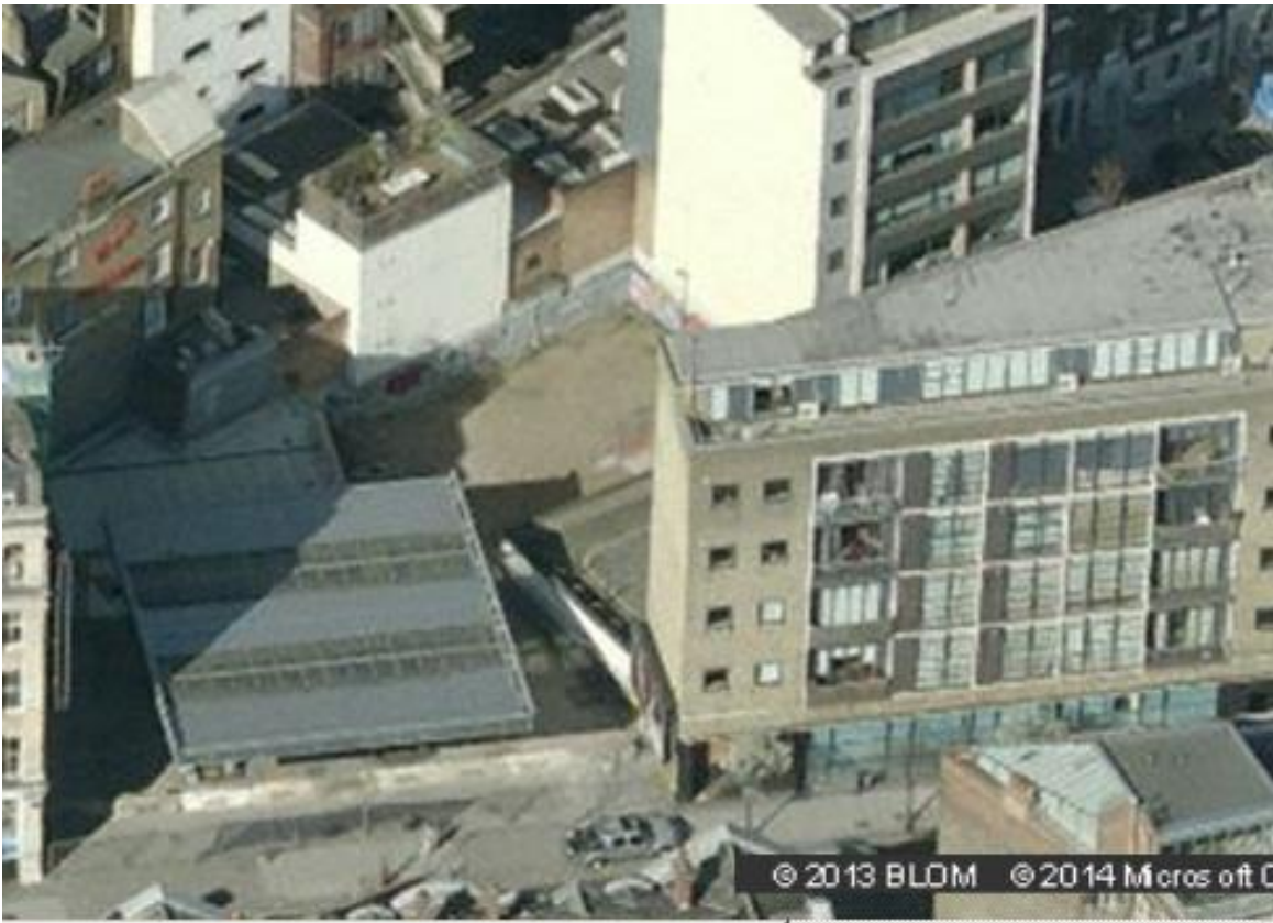
Image 1: Aerial view northwards into the application site
